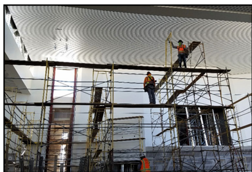
Installing the ceiling in the Church
