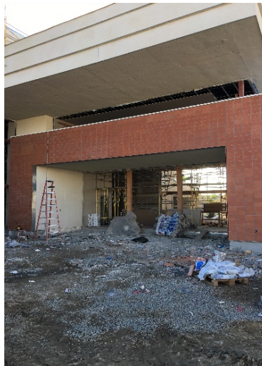
Red brick on Church entry
