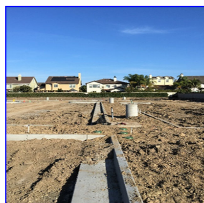
Parking lot curbs and planters
