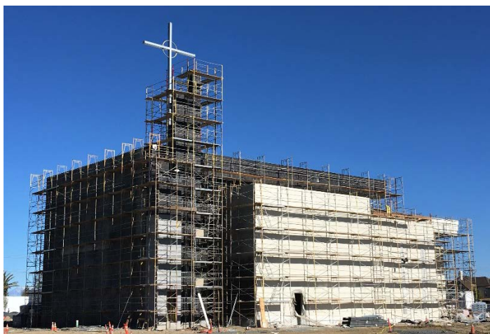
South wall of Church is being plastered
