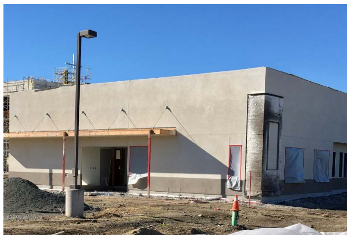
Exterior of Parish Center has been painted
