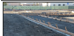
Turn-about entering from main entrance to property from Raitt.
