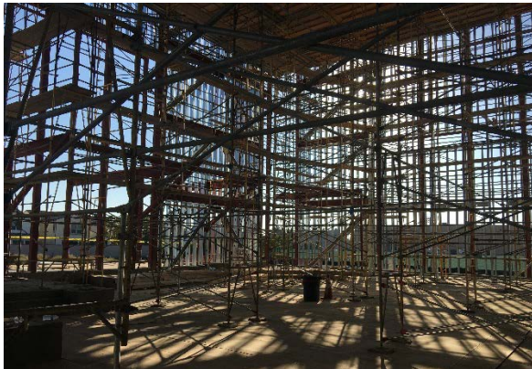
Scaffolding inside the spacious Church
