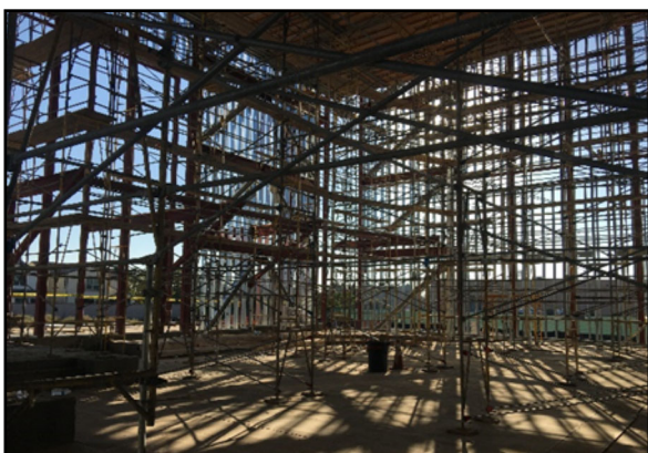
Scaffolding inside the spacious Church
