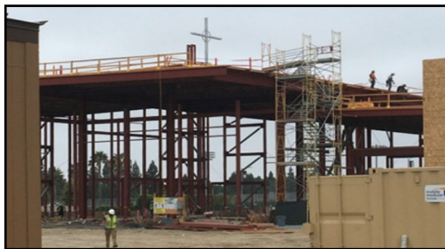
The roof is secured on the new
