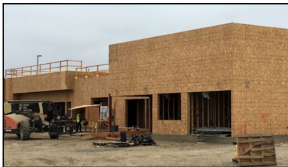
The Parish Center is taking shape inside and out
