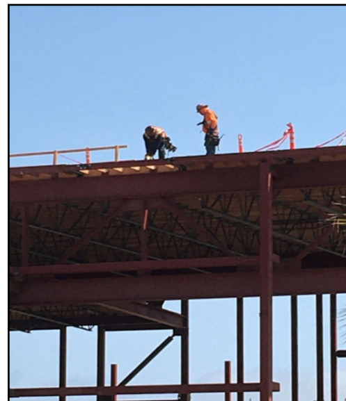
Construction teams working at high altitudes
