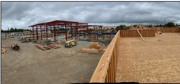
A VIEW FROM THE ROOF OF THE PARISH OFFICE TOWARDS THE SANCTUARY OF OUR NEW CHURCH.
