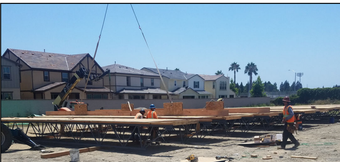
PREPARING THE JOISTS FOR THE ROOF OF SANCTUARY OF NEW CHURCH.
