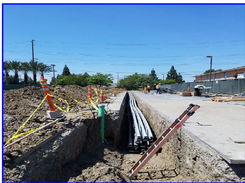
Providing electricity to the new building
