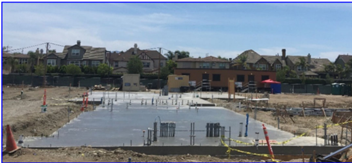
The foundations have been poured . . .
