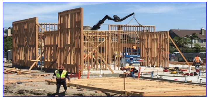
Framing for the Parish Center has begun . . .
