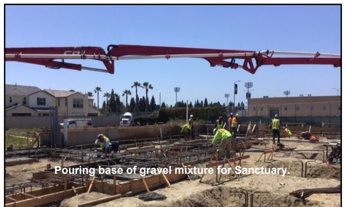
Bayley Construction Superintendent supervising pour of concrete foundations for pile caps/steel columns for Sanctuary.
