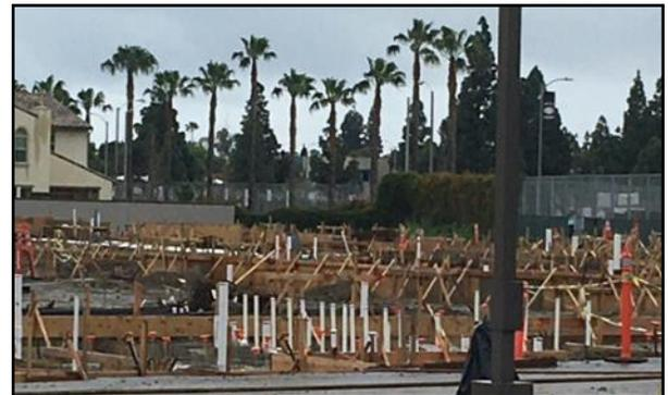
*Now that the underground utilities are in place.....forms are being built for the foundations of the Church & Parish Center.*
